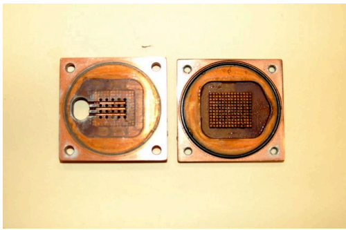
Inside the heat exchanger. Note the lint build-up on the right side.
