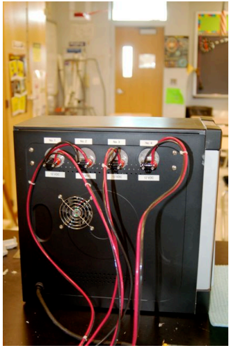
Modified computer case with power supplies inside.
